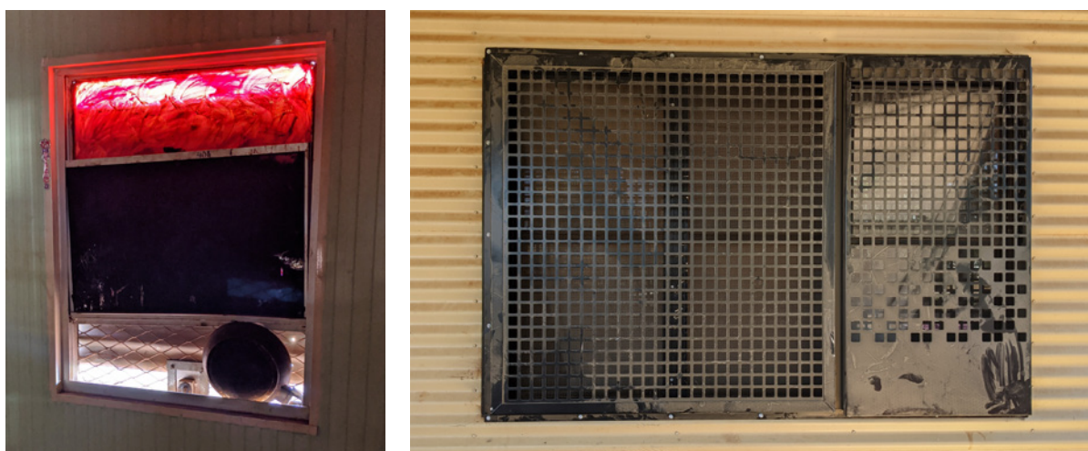
Figure 12: Window and window security screen, APY Lands
