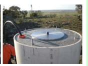
Figure 4: Construction of the GNSS CORS pillar plate at a CORSnet-NSW site
