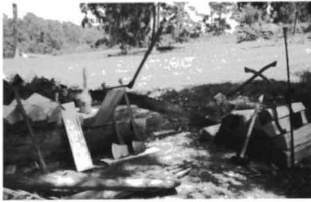
Figure 39. Shingle splitting tools and split shingles.
