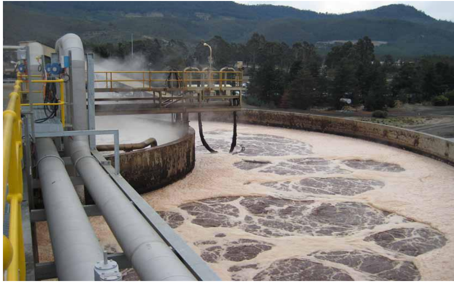
Figure 2.1: The NSB SETP. The inner holding tank is the biofilm reactor (BFR) and the outer tank is the activated sludge reactor (ASR).
