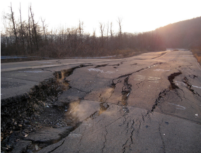
Fig. 3. Subsidence along the abandoned Route 61 highway due to the underground coal mine fire in Centralia, USA. Photo: Angela Parriott.
