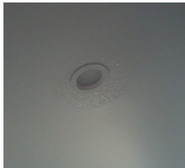
Fig. 2. Condensation forming around downlights.
