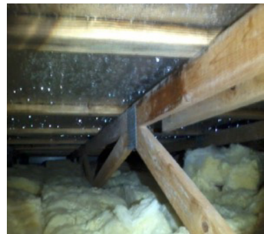
Fig. 3. Condensation forming in roof space.
