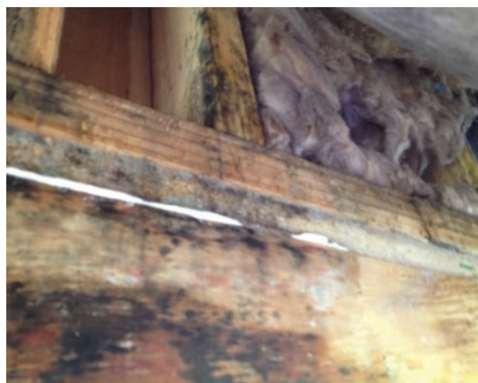
Fig. 8. Mould growth on bearer, joist, wall batts and gaps left in wall insulation.
