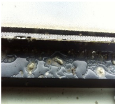
Fig. 1. Excessive condensation and mould on aluminium window.
