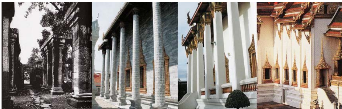
Fig. 25: The evolution of bracing projecting roofs in traditional Thai temples and palaces From left to right; the columns of Phimai Palace, built in 12 th century; exterior columns at Rachapradit Temple; the combination of tapering redented columns and eave brackets at Daowadeungsaram Temple; and bracketed construction in serpentine shape at Dusit Throne Hall. (Sthapitanonda 2006, p.125 & 160)
