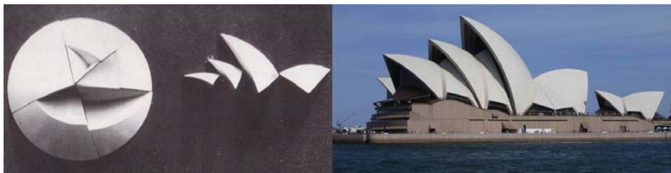
Fig. 22: The modern adoption of multi-tiered roofs in Australia is conspicuous in The Sydney Opera House (1975), designed by the Danish architect, Jorn Utzon (1918-2008). The spherical geometry of the individual roof vaults actually came from a segmented orange, not from white sails. (Drew 1995, p.14) and (Kongsuwan 2005)
