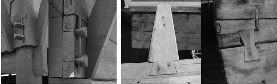
Fig. 29: Butterfly and dovetail joints in traditional Thai joinery
