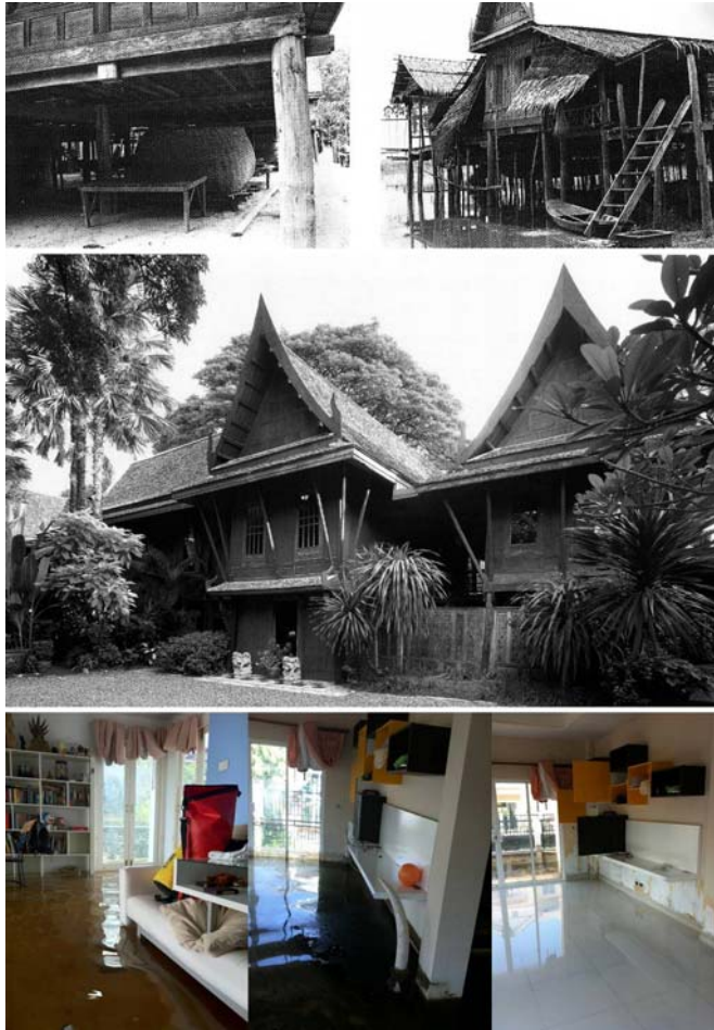
Fig. 3: The top row shows the raised floor of traditional Thai houses protecting the house from flooding (Chaichongrak 2002, p.48); The middle row shows the hybrid function of the ground floor of Jim Thompson's Neo-traditional house 2 which was adapted according to Western functional utility (Sthapitanonda 2006, p.239); The bottom row shows the damage on the ground floor of modern houses and built-in furniture during and after flooding in 2011, Nonthaburi, Thailand. (Kongsuwan 2011)
