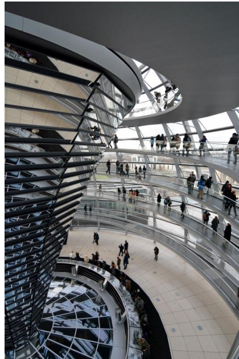
FIGURE 6.25 The dome's interior, with conical ventilation and light reflecting device, and, at its base, the observation windows into the plenary chamber beneath.
