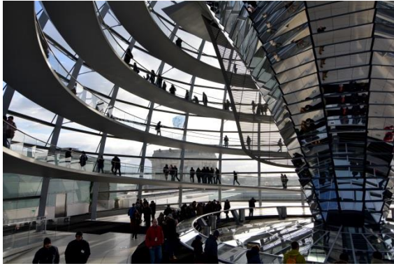
FIGURE 6.26 The dome's double helix ramp system for ascending and descending the dome.
