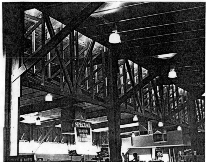
Plate 3.10 4.80 metres high laminated veneer lumber trusses running through glu-laminated twin portal frames in the hardware wing.
