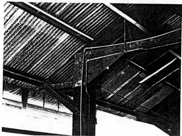
Plate 1.68 Detail of bottom chords connected to 50 x 150 mm solid hardwood timber column. To strengthen the jointing, mild steel gusset plates 4 mm thick connected using M 20 bolts are used.
