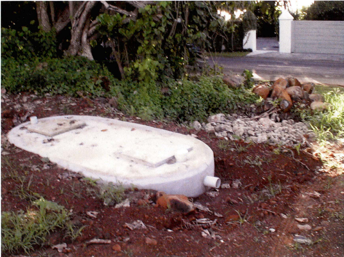
Figure 4.3 A recently installed Cook Island Health Department approved 2000L concrete septic tank and overflow soak hole.
