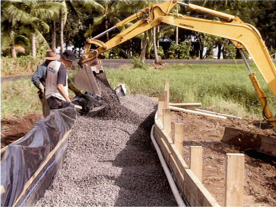
Figure 4.10. A local back hoe carefully places the core treatment zone prescribed material without damaging the base liner
