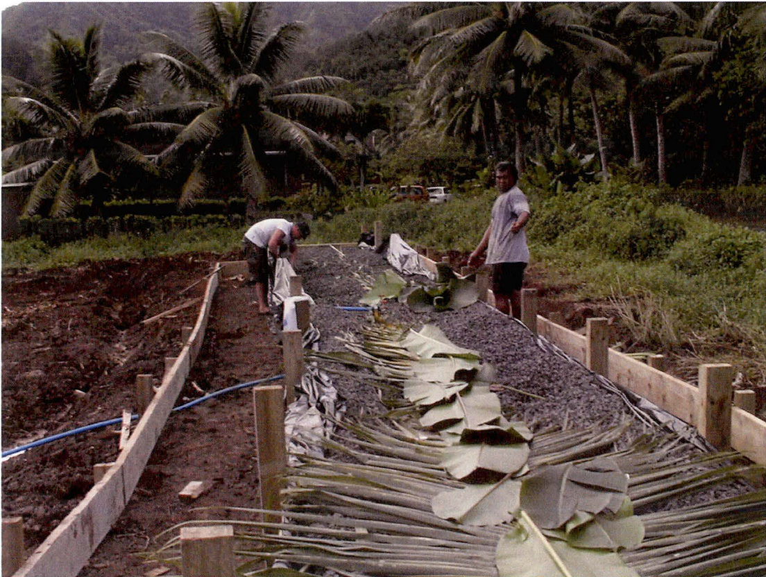
Figure 4.11 Locally available materials such as coconut fronds and banana leaves used instead of geo-textile fabric
