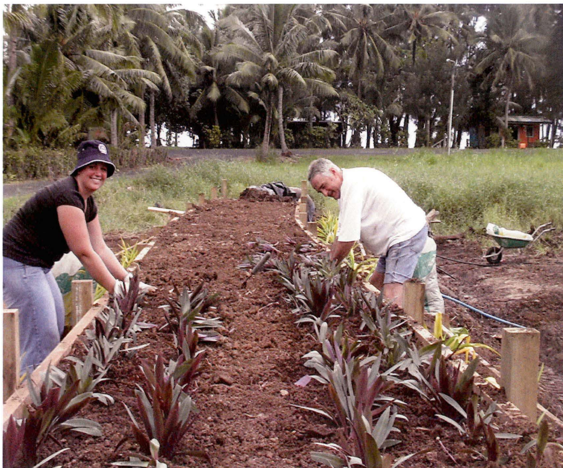
Figure 4.12. Selected drought tolerant plants were used to complete the Evapocycle evapotranspiration irrigation areas
