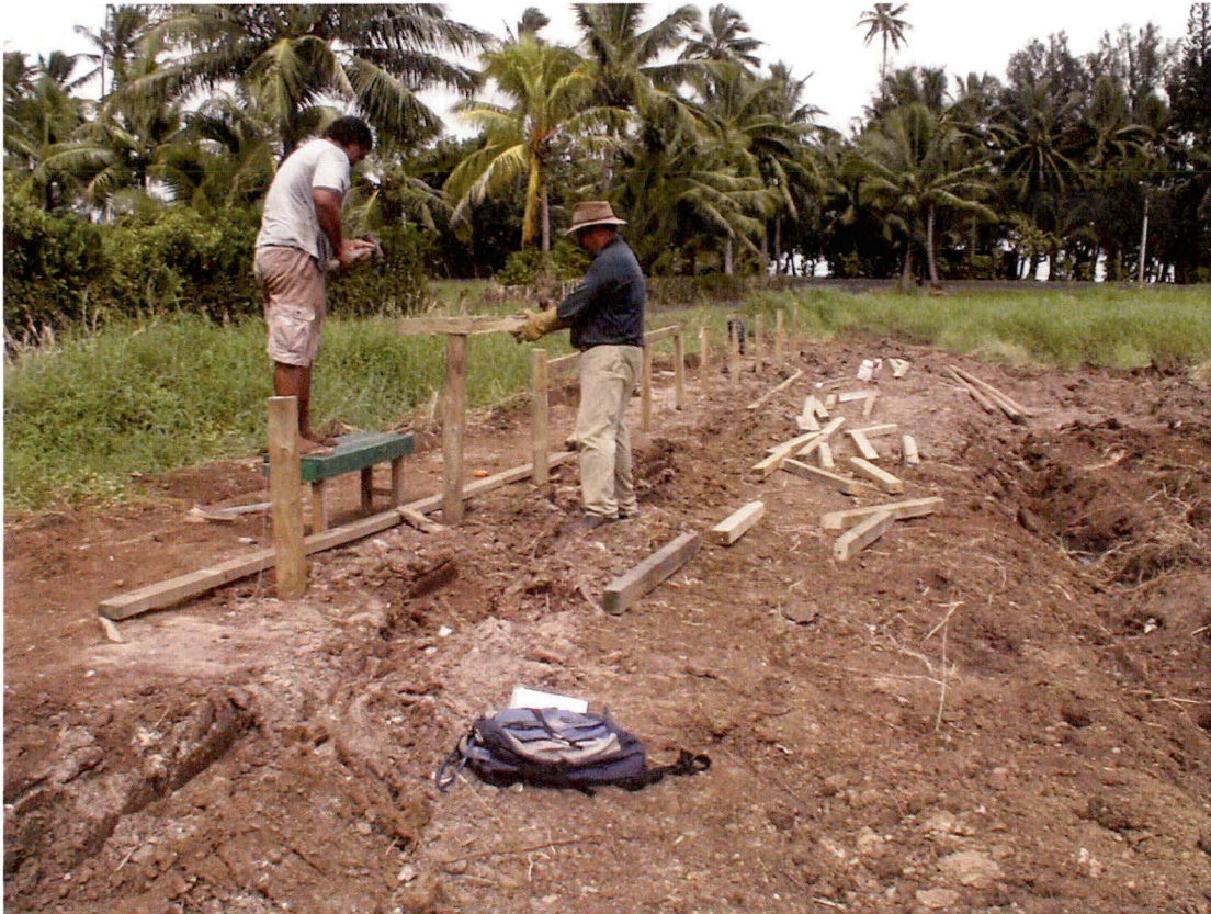
Figure 4.9 Showing locally manufactured treated timber being positioned to support the Evapocycle Core Treatment Zone
